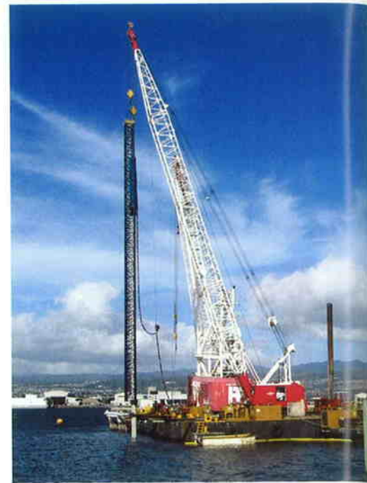
Watts-Healy Tibbitts joint venture conducting test pile driving at Beckoning Point
