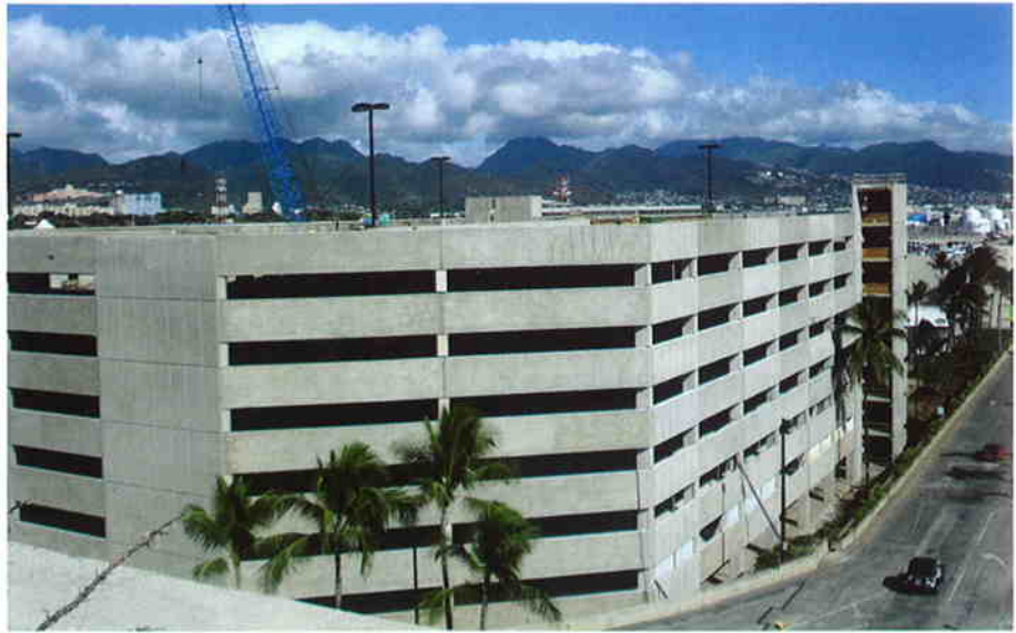
The newly completed eight-story parking structure at Honolulu International Airport. dck pacific construction LLC (formerly Dick Pacific) completed the project.
